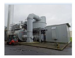
Volatile organic compounds from the extrusion department are burned in a Thermo-Reactor. The hot flue gases are recovered for steam generation.
